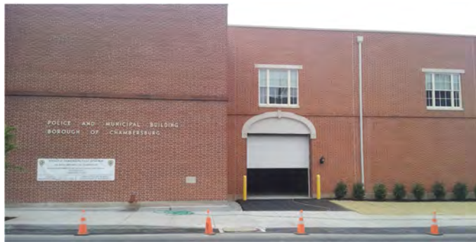
Newly completed addition to the Police Station and Sally Port driveway
