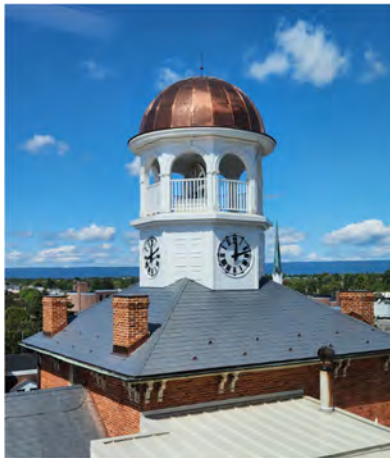
Fully restored Market House cupola and clock tower
