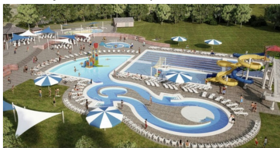
New Memorial Park Pool under Construction in Chambersburg
