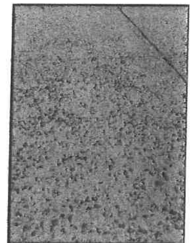
Spalled Sidewalk
