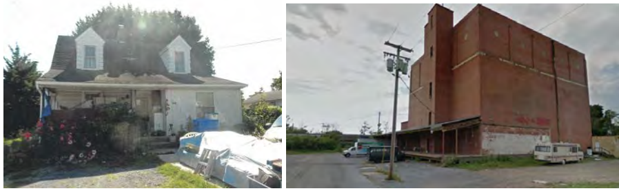
Former Buildings Demolished
