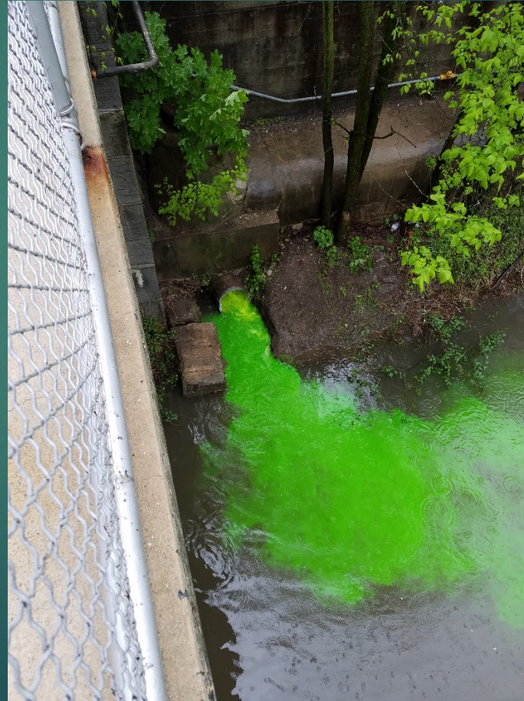
AFTER PIPE LINING
