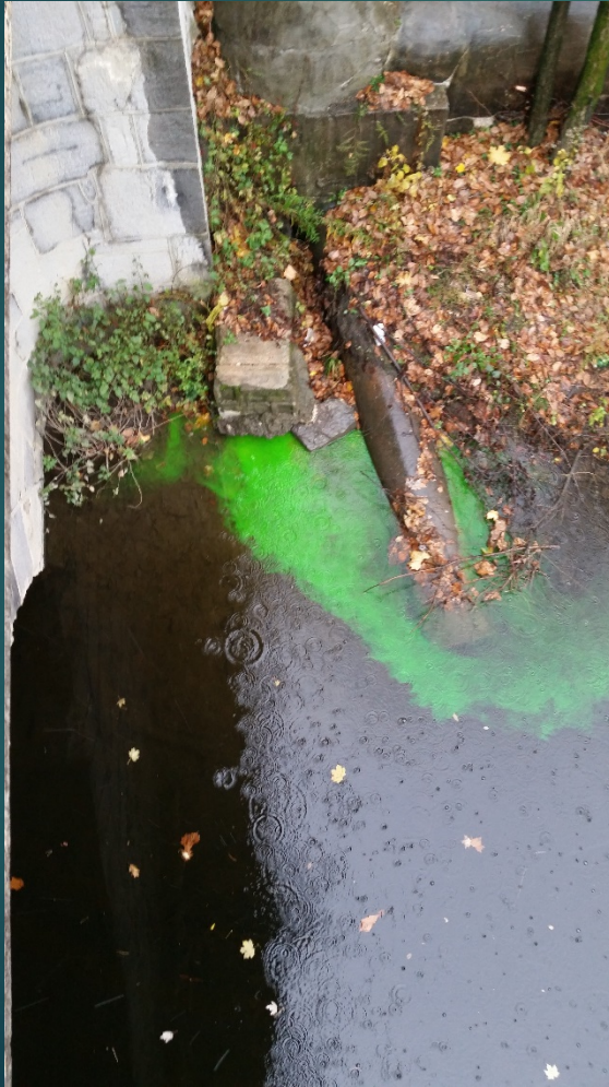
BEFORE PIPE LINING
